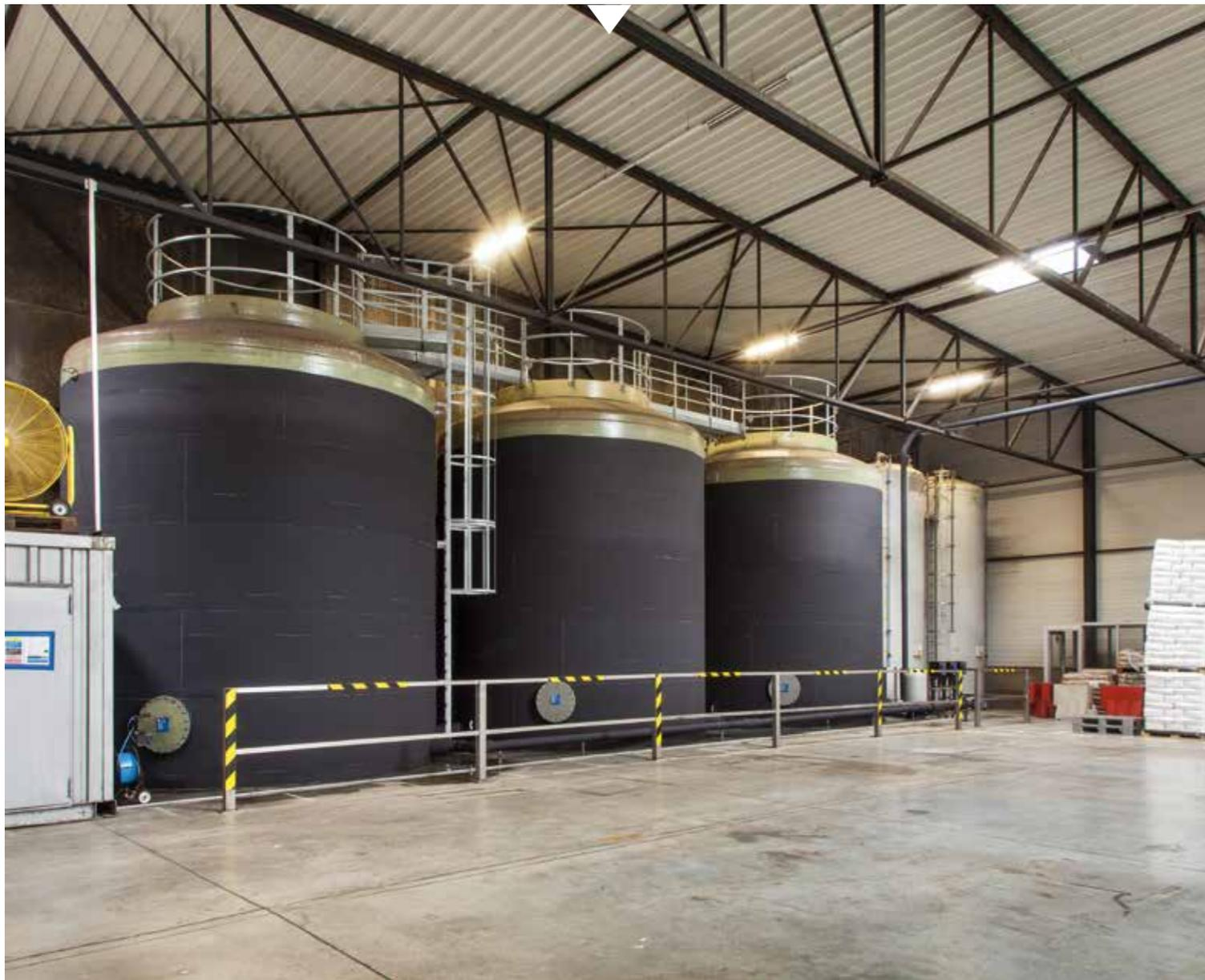
Our GRP or polyester tanks have an excellent resistance to chemicals and excellent mechanical properties. This makes them the ideal solution for aggressive and corrosive environments and underground tanks. Applications can be found in the chemical industry (HCl, NaOH), the petro-chemical industry (fuels) and water purification plants (FeCl<sub>3</sub>, sludge). Moreover, polyester tanks require little or no maintenance, are not conductive and are unaffected by stray currents!
